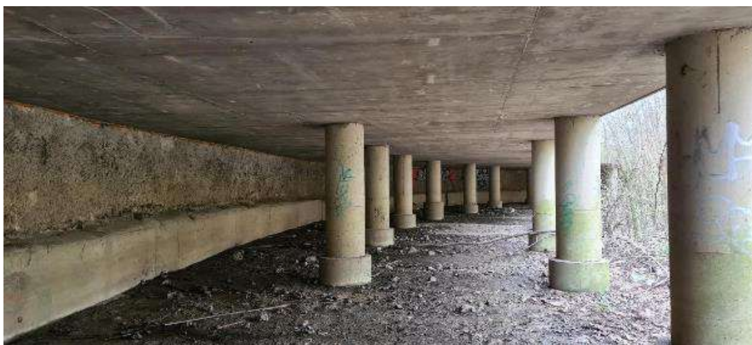
Figure 13: View from the stilt structure supporting Longbridge SLTL
