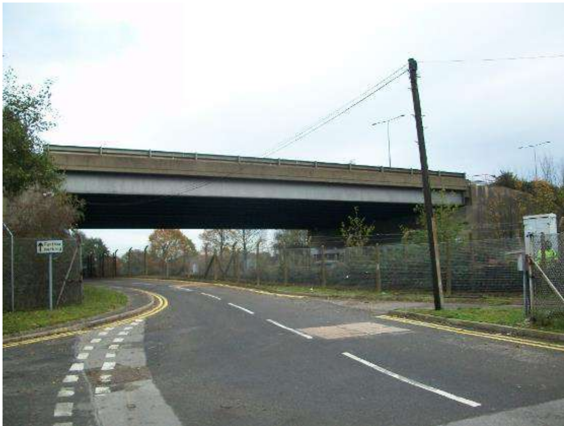
Figure 23: Existing Airport Way Bridge
